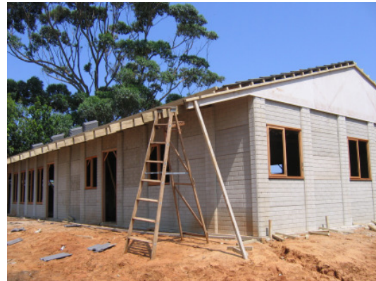
Youth Centre under construction Nov 2007
