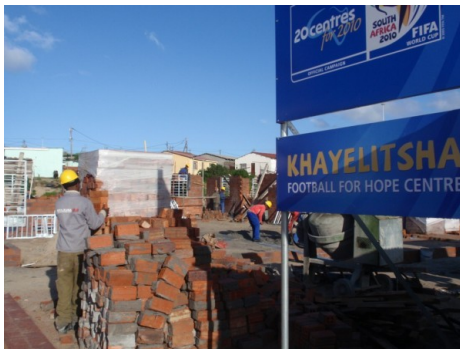
The Football for Hope Centre under construction
