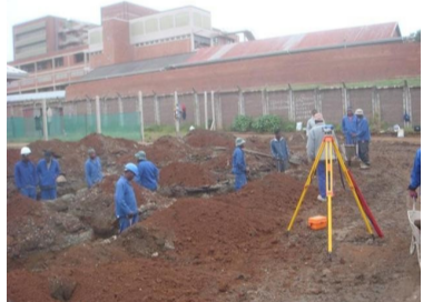
Foundations being dug for the new Health Academy
